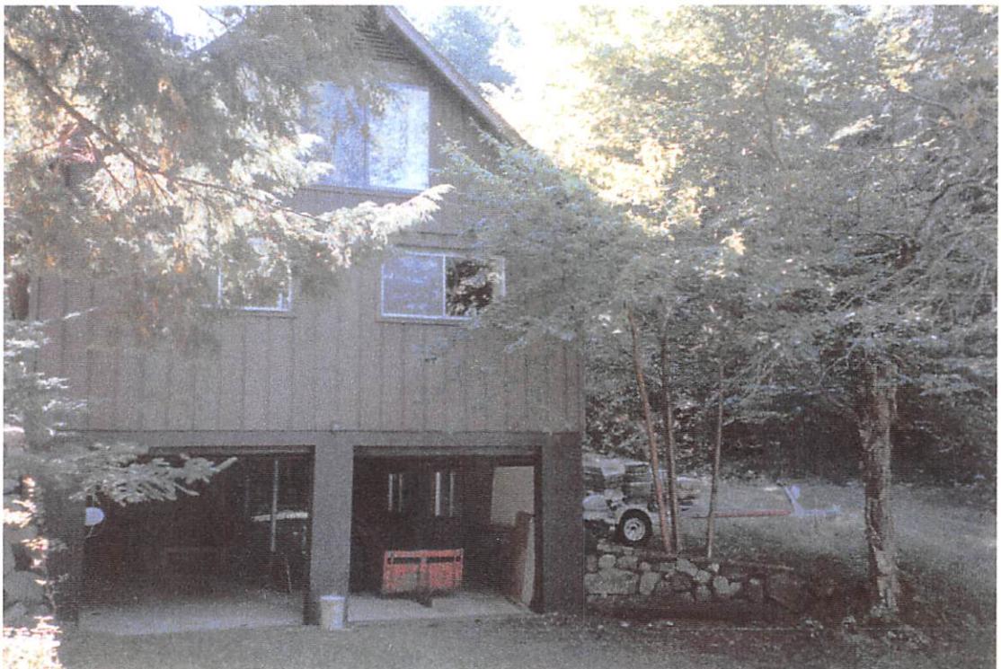
Lower Level of Garage
